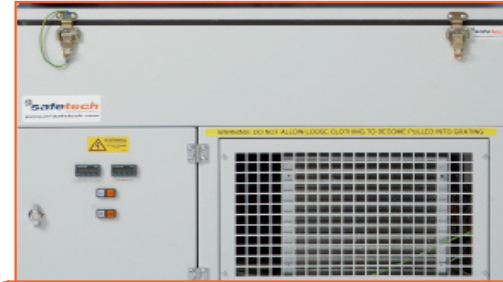
The hand built air treatment unit sits at the core of the ClimateZone operation, regulating both temperature & humidity.
